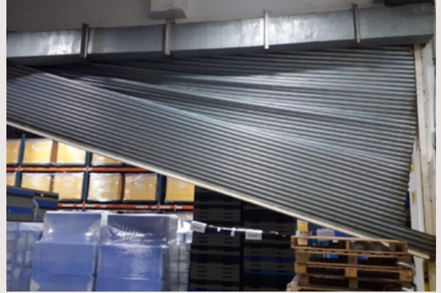
STUCK & JAMMED SHUTTER
