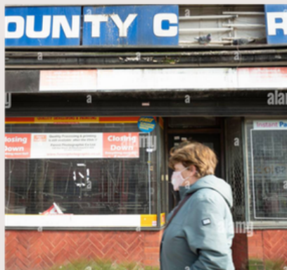
SHOP SIGNS BOARD REPAIR
